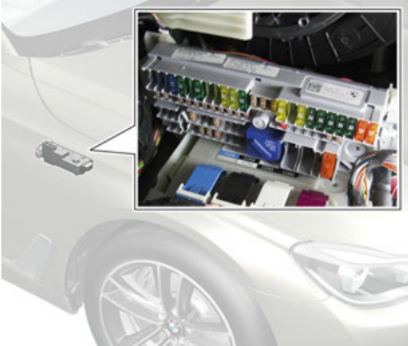
Power distribution box, front right
